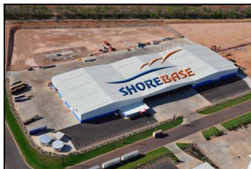
ShoreBase Operations at Hudson Creek
